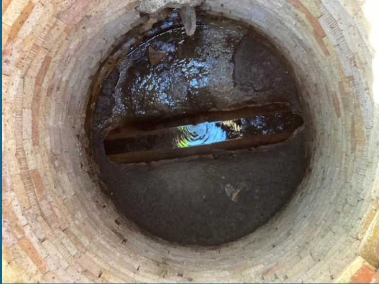
Before manhole rehabilitation
