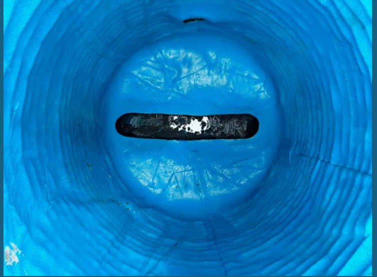
After the CIP Liner is installed
